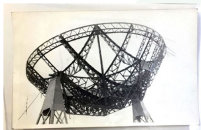
The paraboloidal dish of an ex-WWII German Würzburg 7.5m radar, used by Ryle (photo credit: Churchill Archives Centre).
