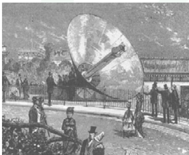
In 1878, Augustin Mouchot constructed a printing press that ran on steam generated by a solar thermal collector. See https://commons.wikimedia.org/wiki/File:Mouchot1878x.jpg . Public domain, via Wikimedia Commons.
